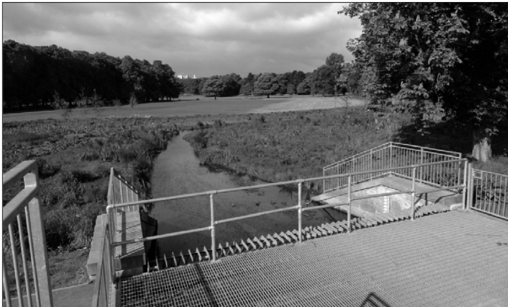
Figure 3. Inch Park Flood Storage Reservoir from the Outlet Structure
