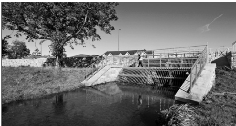
Figure 4. Inch Park Flood Storage Reservoir Outlet Structure
